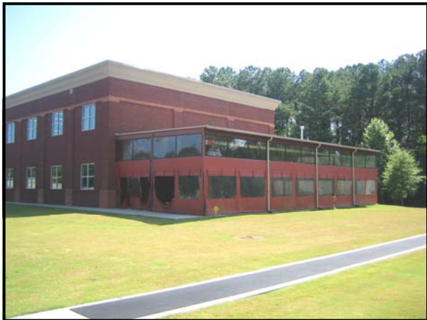
Enclosed & Covered Patio
