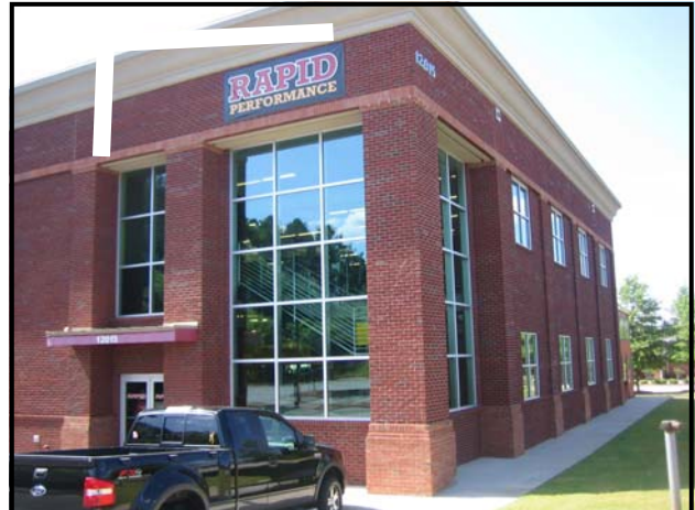
Close Up of Front Entrance
