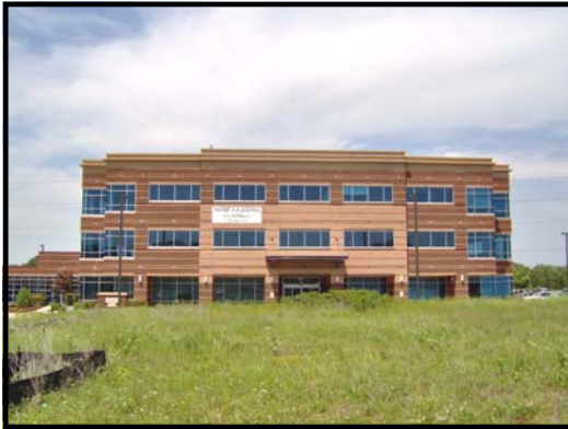
Front of Building
