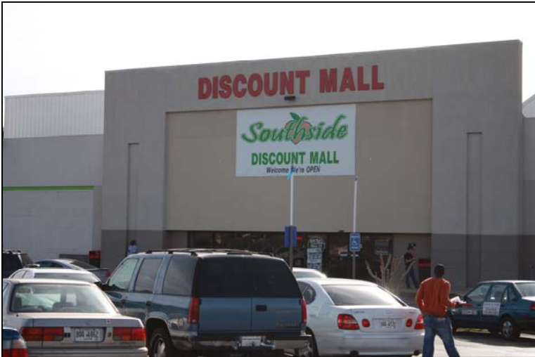
Front of Property
